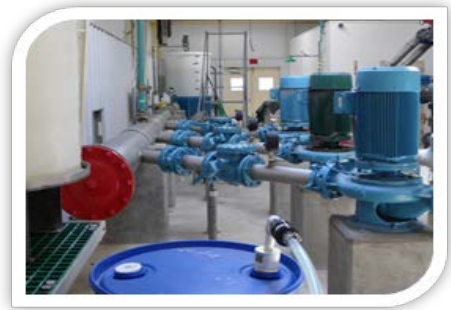
FIGURE 5.3.8 FINISHED WATER PUMPS
