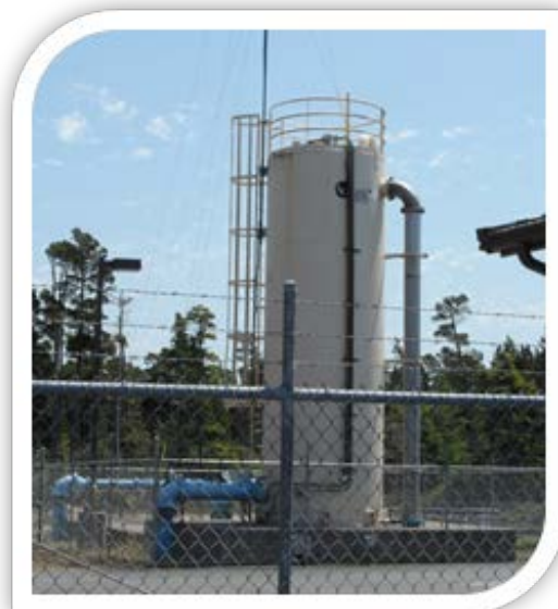
FIGURE 5.2.1 RAW WATER SURGE CONTROL TANK
